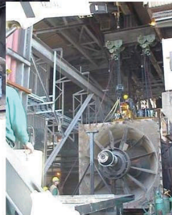
Photos show maintenance of ID fan & rotor at a local power plant
